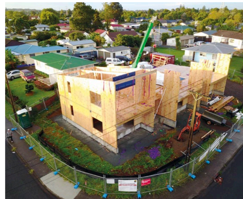
Everitt Road, Otara
